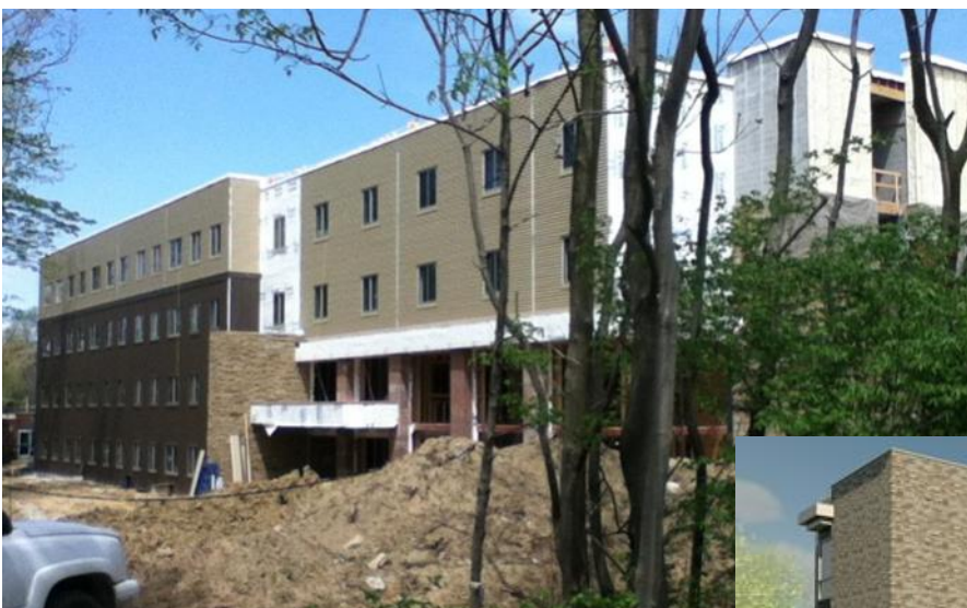
Recent Construction Photo
